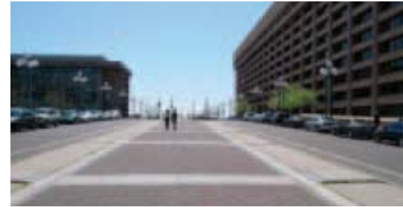
These buildings and streets are exceedingly out of scale for pedestrians.
