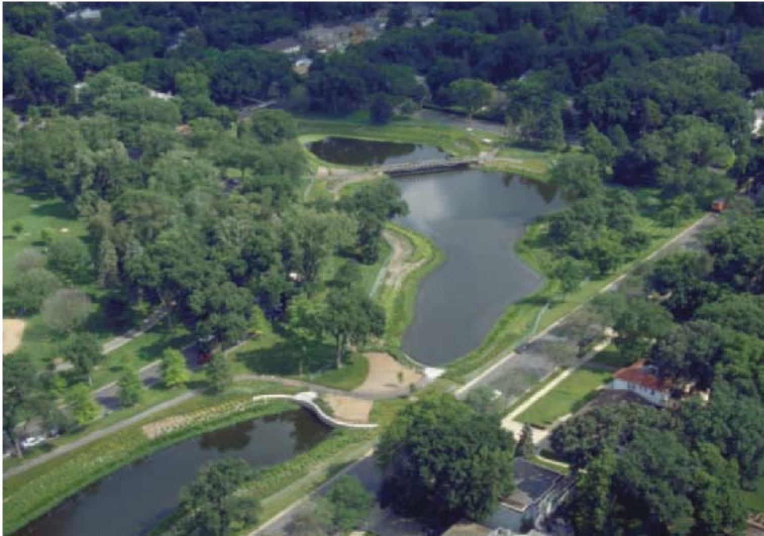
A project of Minnesota's Chain of Lakes Clean Water Partnership, the Lake Calhoun constructed wetlands and ponds in Minneapolis improve water quality by intercepting storm water runoff and filtering out pollutants and sediment.
