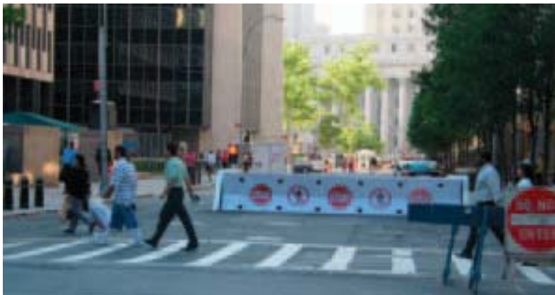
Concrete barrier limits vehicles at Federal Plaza, Duane Street, Lower Manhattan, N.Y.
