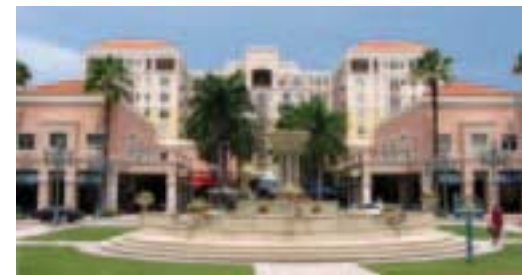
Mizner Park in Boca Raton, Fla., is one of the most successful mixed use, infill redevelopment projects in the United States.
